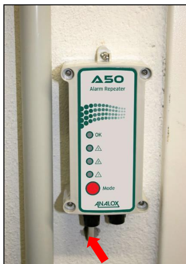
Repeater connections (Hard wired shown)
